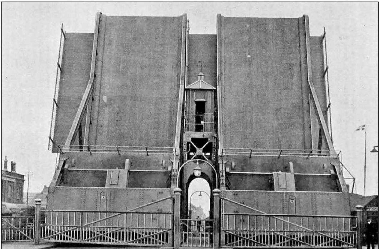
1913 view to east from City end with both bridges lifted. The two counterweights now form a barrier to road traffic in addition to the gates. Note also the housings for the motor and gears on the platform in front of the counterweights. (Griffith 1913)
