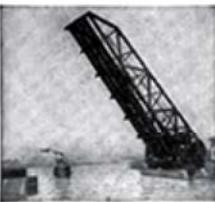
Scherzer Rolling lift bridge—Partly Open.
