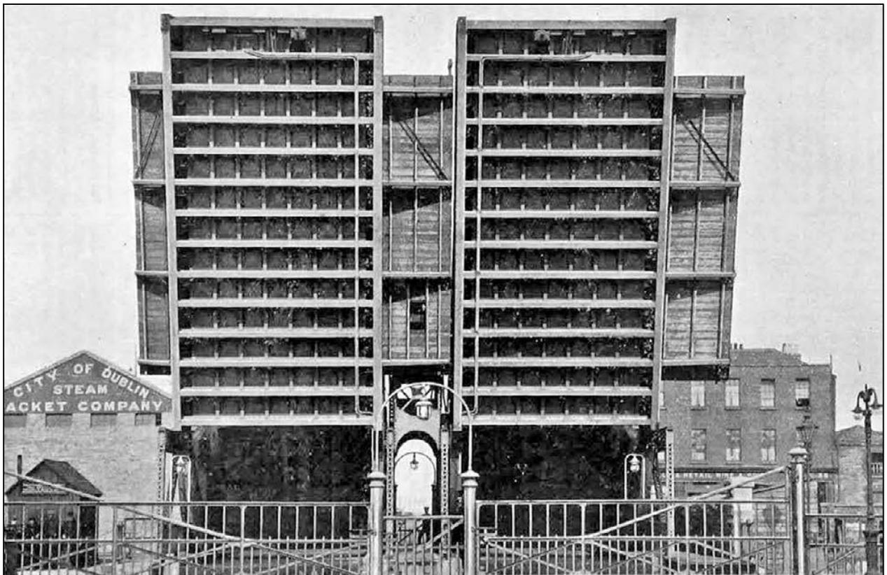
**1913** View from west towards City end showing both bridges raised to permit boats to pass through underneath. (*Griffith 1913*)
