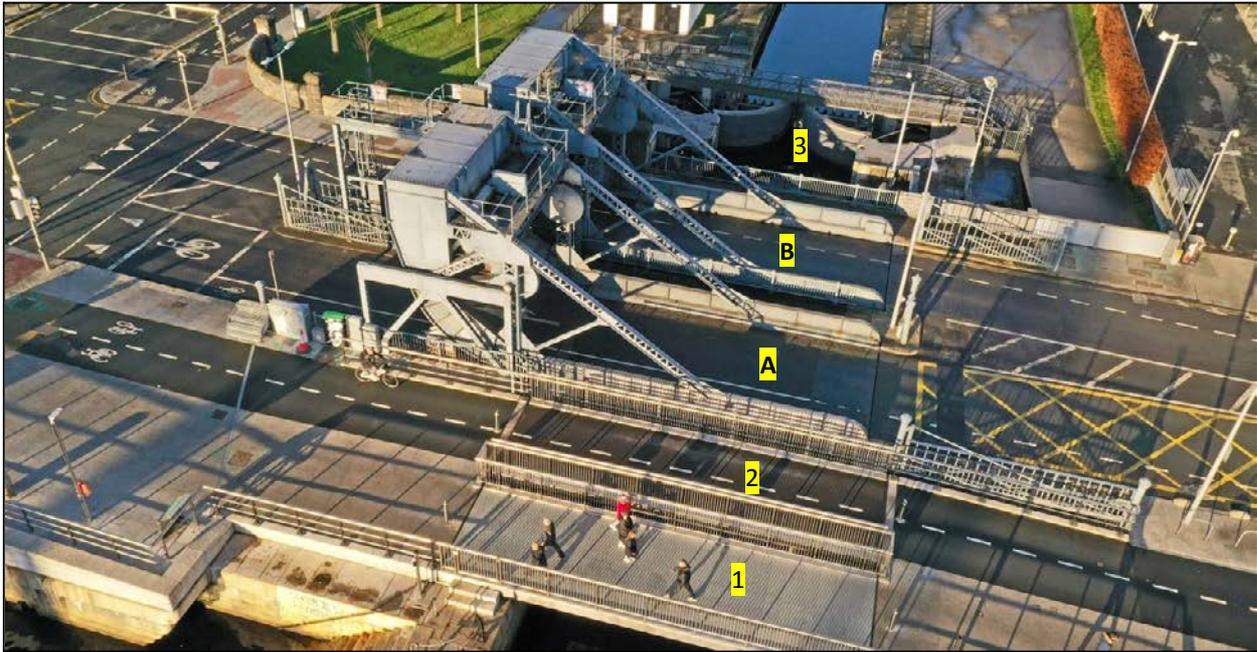
Fig 3.11 Aerial view of modern bridges over the Royal Canal from south, 2021. Key: A - Outer Scherzer; B - Inner Scherzer; 1 - 2019 foot bridge; 2 - 2019 cycle bridge; 3 - Bottom lock gates/ flood barrier.
