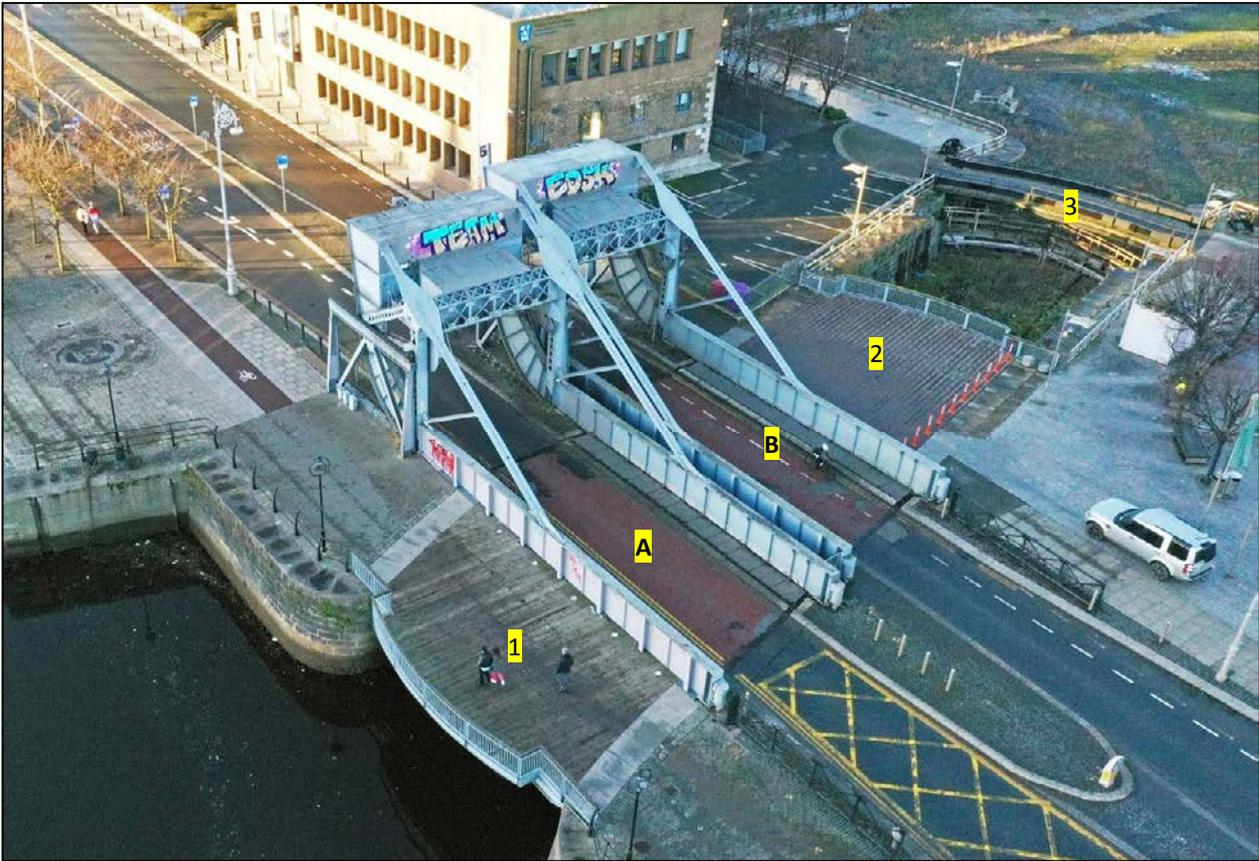
Fig 6.9 Aerial view of modern bridges over the entrance to George's Dock, from SE, 2021. Key: A - Outer Scherzer; B - Inner Scherzer; 1 - Modern foot bridge; 2 - Modern footbridge; 3- Vehicle access bridge.
