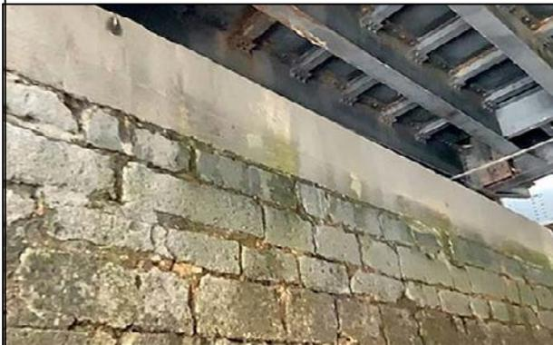
Outer Bridge showing concrete pillow block along top of masonry side wall of canal. This replaced several removed courses of stonework.
