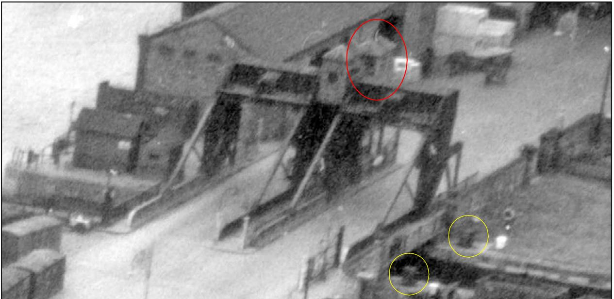
Enlarged aerial view from NE, 1950. The original control cabin platform has now been extended towards the City end and a second cabin erected (circled in red). Note also the two winches (in yellow) which were installed to work the timber lock gates when the Inner Bridge was erected. They still exist but are no longer in use. (*Britain from Above, XAW032929*)
