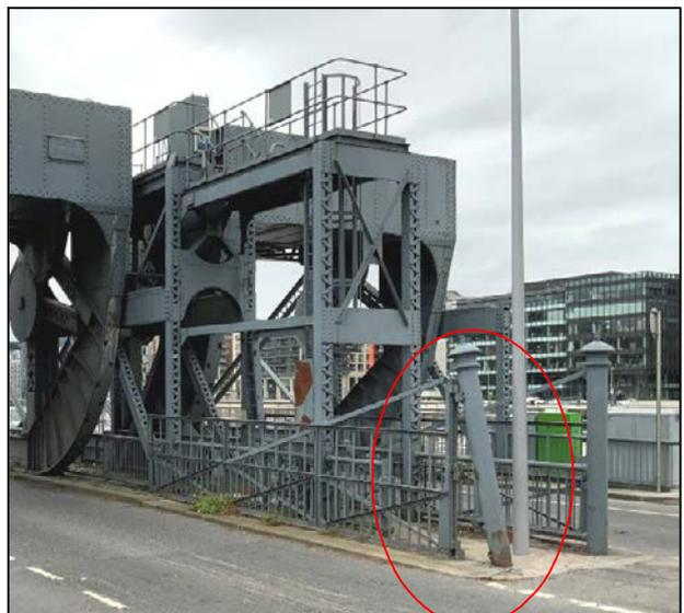
Fig 4.5 Traffic impact damage. *Left*: Bent flange on main girder at east end of Outer Bridge. *Right*: Damaged traffic control gatepost at west end of Inner Bridge.
