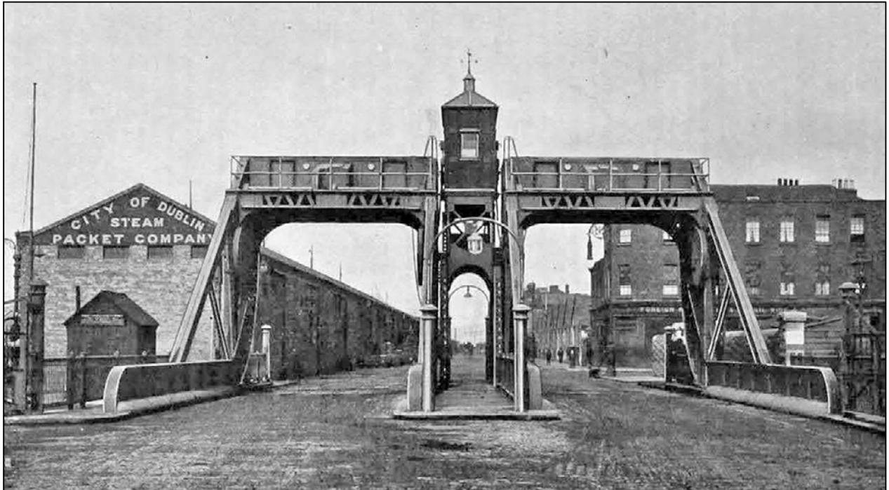
**1913** View from west towards City end showing both bridges open for road traffic. The motors which powered each of the bridges is visible half-way along each gantry in front of the overhead counterweights. (*Griffith 1913*)
