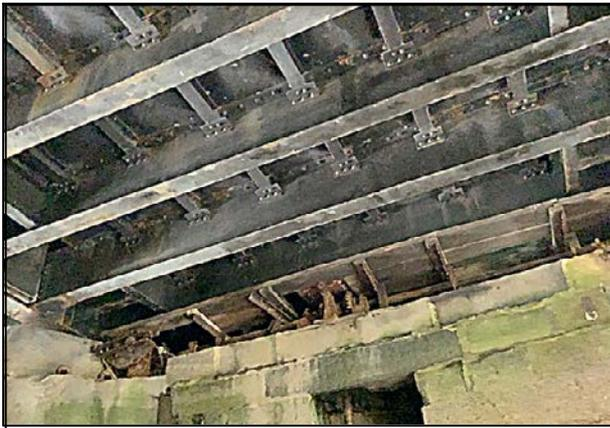
Inner Bridge showing the lock gate operating linkage along the top of its gate emplacement. The gates were operated using winches just beyond the bridge.
